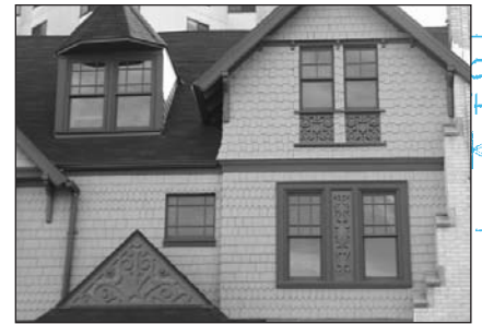
Pozzi Wood Windows grace the front of Peck Row Condos, replicating the look of the original 1883 windows.
