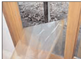
Builders save about $600 per home in clean-up costs by installing windows with protective film.
